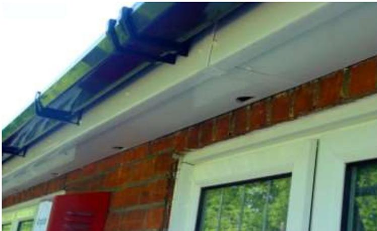
Plastic soffits that have been fitted with internal partitions and drilled with Starling-proof entrance holes for the Swifts to gain access and make their nests inside. These soffits are isolated totally from the roof interior
