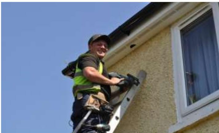
A specially trained workman cuts the right size hole in the right place to let Swifts back into these eaves, where they have been nesting already for many years, after the fitting of new soffits and gutters.
